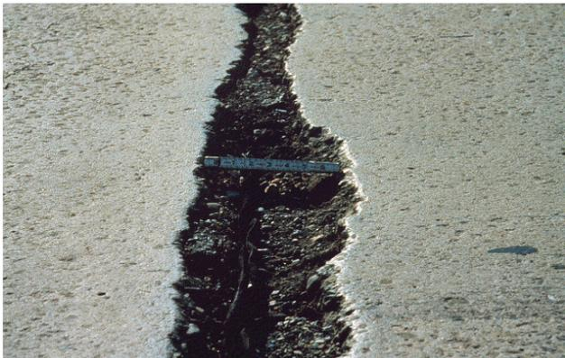
Figure 132. Deck spalling along joint. Location 2.
