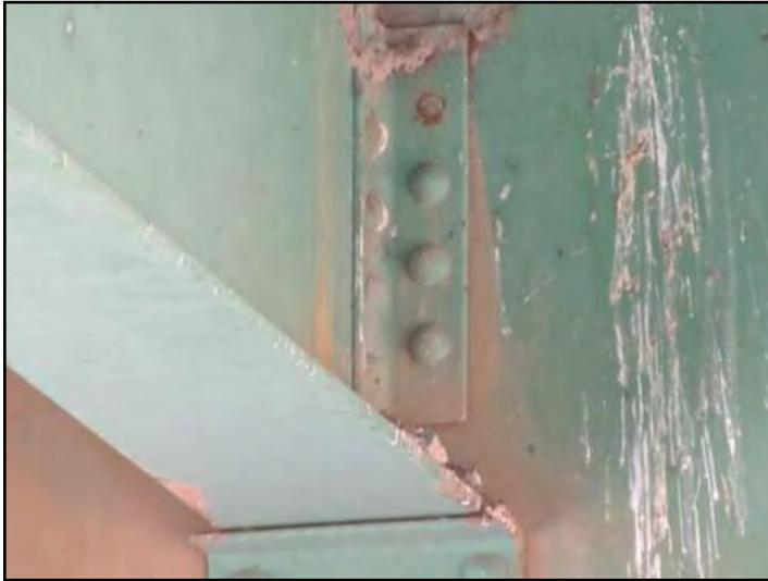
Figure 136. Missing rivets in stringer-to-floor-beam connection. Location 4. (Source: Colorado DOT)
