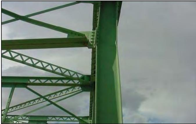
Figure 135. Distortion in truss vertical. Location 1. (Source: Colorado DOT)
