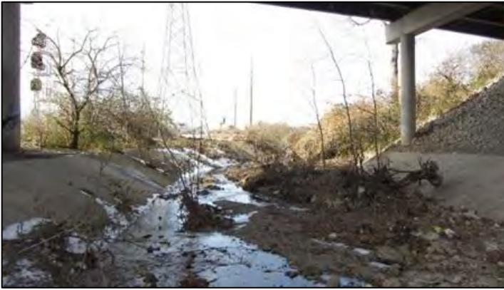
Figure 178. RC lined channel with debris and vegetation for Bridge Number 15558X.
