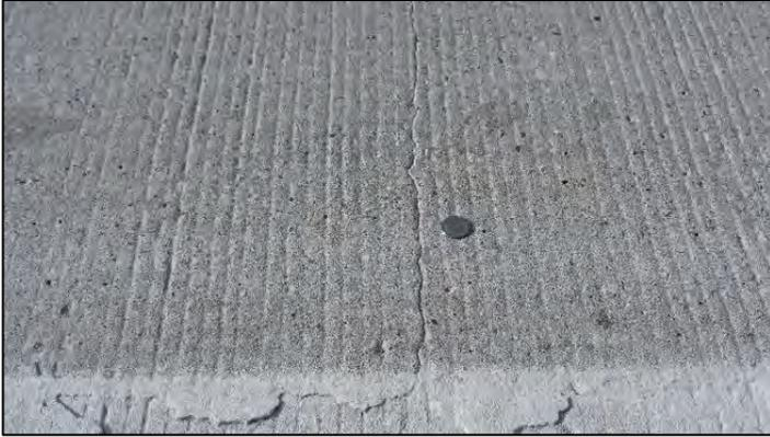
Figure 160. Transverse cracking in top of RC deck for Bridge Number 15558X.
