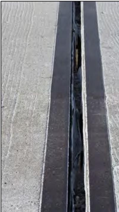
Figure 177. Strip seal ripped and punctured completely through for Bridge Number 15558X.
