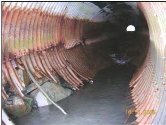
Figure 141. Corroded pipe culvert invert. Location 1 and 3. (Source: Alaska DOT)
