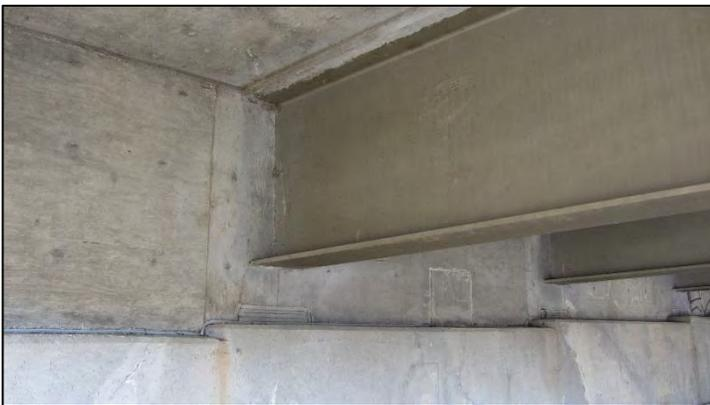
Figure 170. Cracking in north RC abutment for Bridge Number 15558X.
