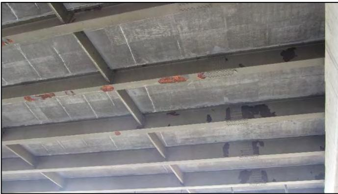
Figure 164. Spot surface corrosion on steel beams for Bridge Number 15558X.
